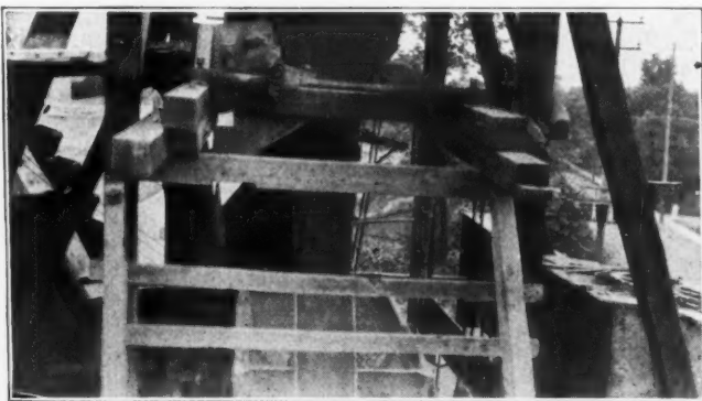
View of Trommel and Screen
